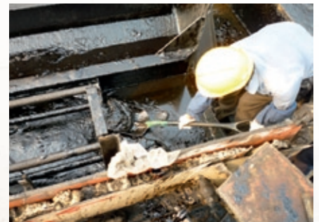
Dirty work – sludge removal by hand.
