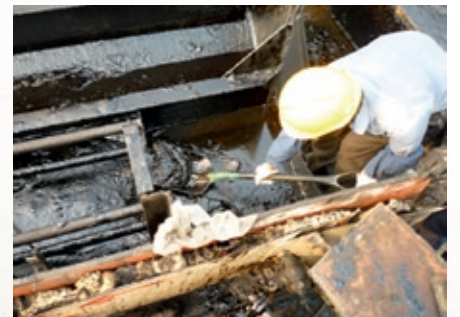
Dirty work - sludge removal by hand.
